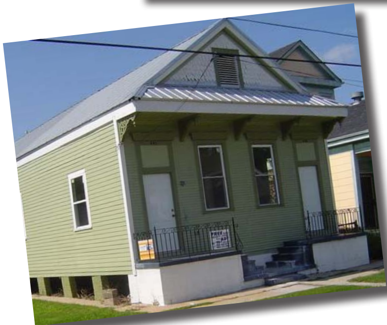
This is the house that Rev. Sally Iberg and the CMA crew worked on in April 2008. It's nearly ready for the three- generation family to move back in
